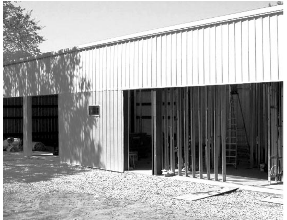
Horticulture/Maintenance Building with Exterior Nearing Completion
