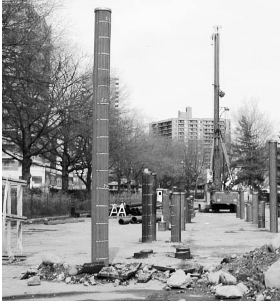
Monotube Piles Being Installed for New Visitor/ Administration Building
