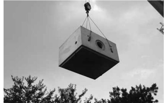
Rainwater cistern section is lowered into place by crane.
